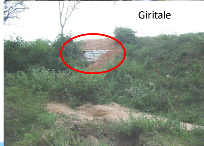
Gated Spillway (Note: Guide wall missing)
